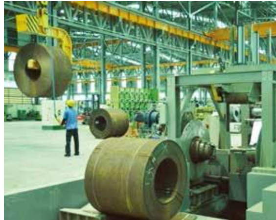
35MT OverHead Crane
