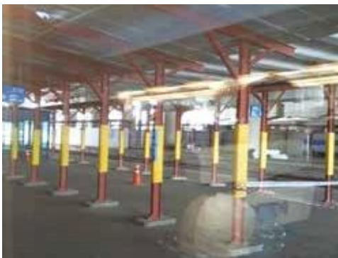
Temporary Support (Recycle) Train Station, Korea H-Beam 150x75x3.2x4.5/6.0
